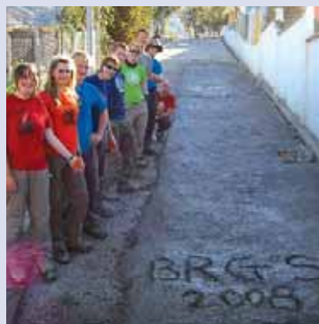
The road built by the team
